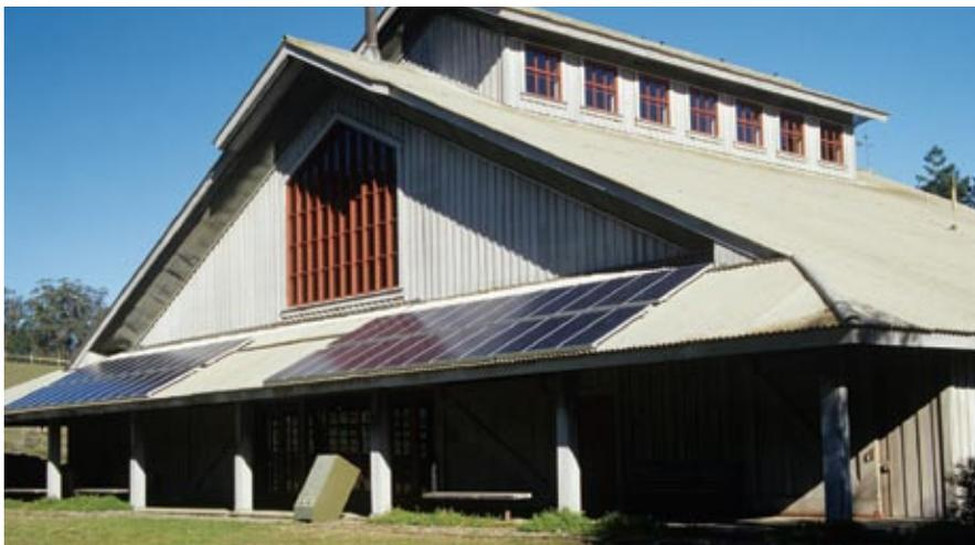
**SUN POWER ON THE FARM:** Use of solar photovoltaic panels, such as those on this barn, is set to become more widespread as clever design makes multicrystalline silicon cells—the most common type—more cost-competitive with conventional power sources.
