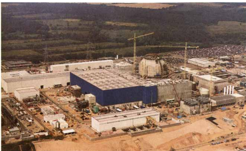
SIZEWELL B will be the first nuclear reactor in the U.K. to contain both conventional and software-based protection systems for emergency shutdowns. Critics argue that the complexity of the software system—it relies on hundreds of microprocessors and more than 100,000 lines of code—makes it difficult to ensure reactor safety.
